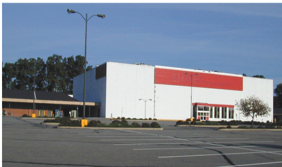
Existing Staples Building-Future Medical Office Building 5/1/03
